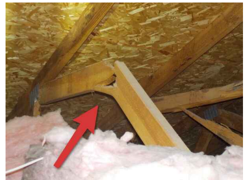
Broken truss
