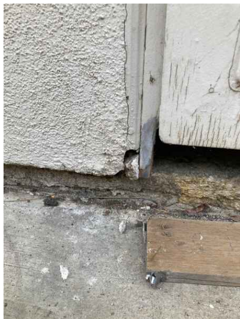
Water heater door
