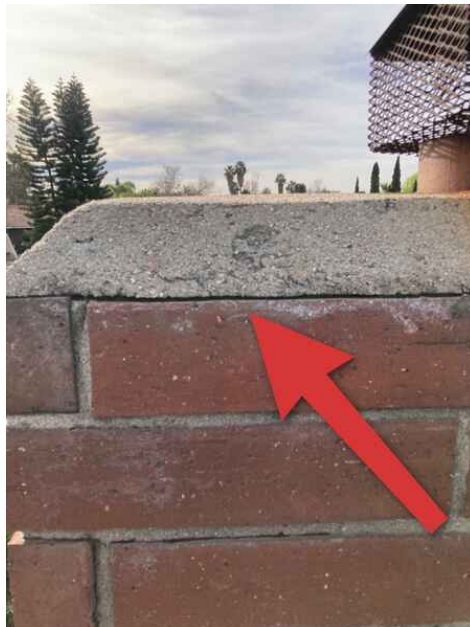
Mortar deterioration
